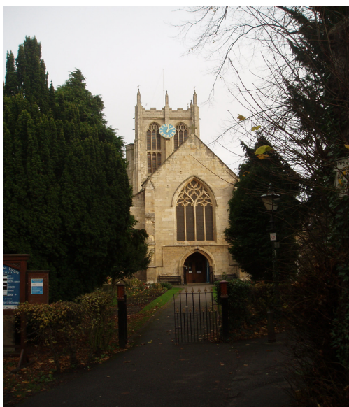
St. Mary's Parish Church, Hallgate (Grade I listed)
